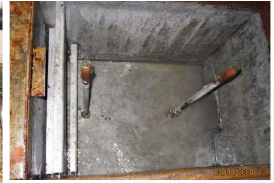
Interceptor pumped out - cleaned to standards.
